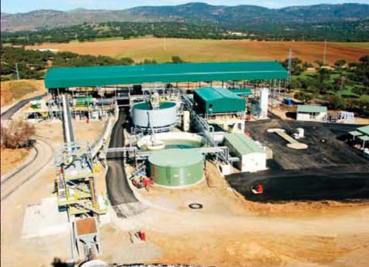
BioMinE Pilot plant Seville, Spain
