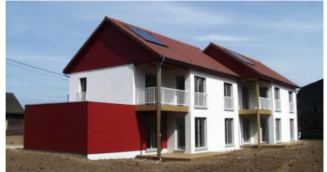
First passive houses in France, Formerie (2007)
